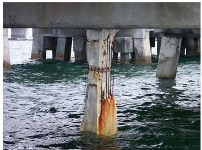
Concrete column damaged by saltwater
