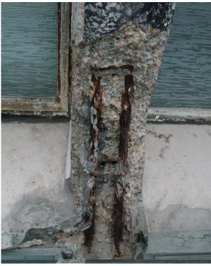
The rust will form Hydrated Iron Oxide (rust) which increases the volume of the steel by up to 10 times its original diameter.
