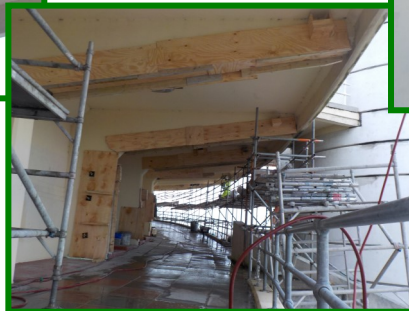
Shuttering around broken out areas ready for repair
