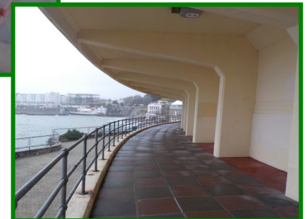
Finished look after Anti Carbonation Coating
