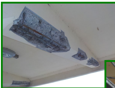
Broken out beam showing corroded reinforced steel
