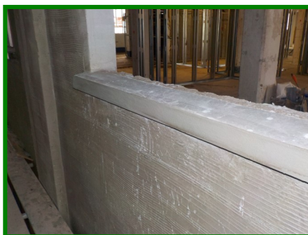
Coating finish to Elevation after repairs where completed using Renderoc ST 05
