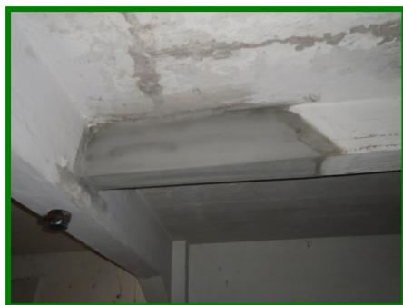
Beam repaired with Renderoc HB45
