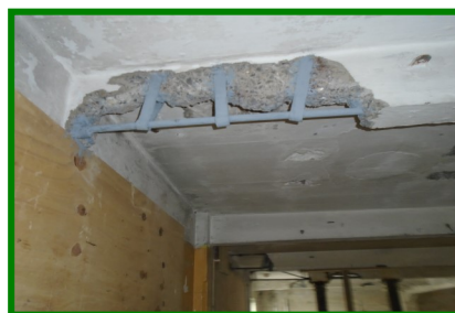
Broken out Beam, steel treated with Nitoprime Zincrich Plus
