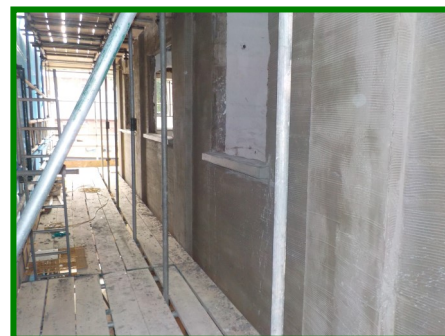
Coating finish to Elevation after repairs where completed using Renderoc ST 05
