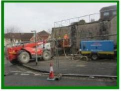
Rock Anchor Fixing - First step was to core drill through the existing wall and then drill through the backfill material and into the rock, fitting the Rock Anchors and grouting the position. The drilling and anchor fixing was carried out using drill rig mounted in a custom built basket on a Tel-Handler with our Subcontractors Saxton Drilling. Cast iron adjustable angel plates were then fitted to secure the wall.
