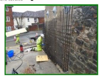
Wall Strengthening - The masonry feature corner and base wall were demolished and removed, the footing excavated around the base of the wall and new foundations laid with steel starter bars. New reinforcement erected and temporary framework fitted. Concrete pours were carried out in phases of 1200mm at a time to ensure the wall strength was uniform and no overloading could occur. FCS Construction (Sub-Contractor) played a key role in the wall strengthening part of the works.
