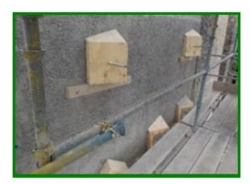
Finishing Works - A new coping details was incorporated onto the last concrete pour and custom built shuttering boxes to form the bearing plates of the anchors were made and poured, followed by render and pebble dashing of the walls to match the rest of the retaining wall.
