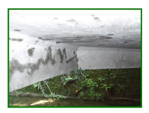
**Defective con**crete around the steel reinforcement being removed to enable cleaning and treatment of the steel.
