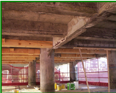
View showing defective beams in the foreground and shutters fitted for re-casting towards the rear
