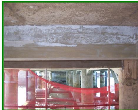
View showing repaired section
