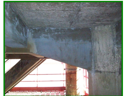
View showing beams prior to repair
