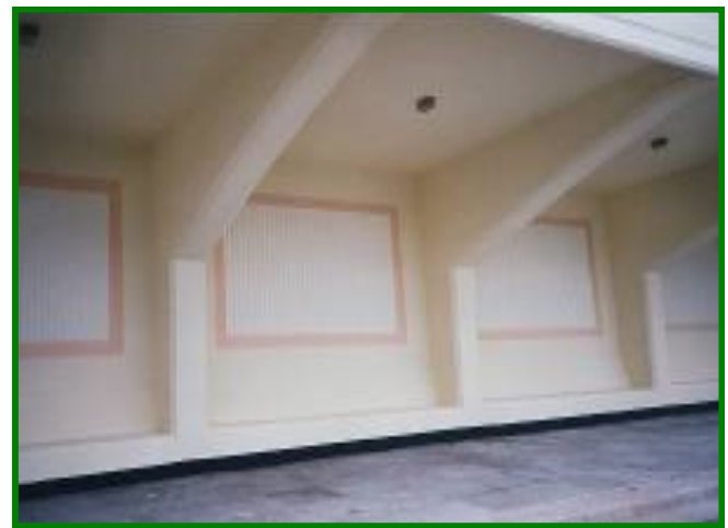
Rear walls showing ribbed feature panels
