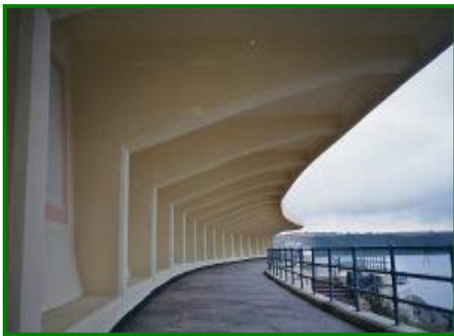
Canopy underside showing structural support
