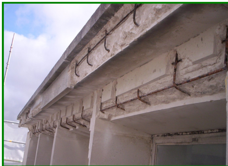
Defective concrete around the steel reinforcement cut away ready for cleaning and treatment of the steel.
