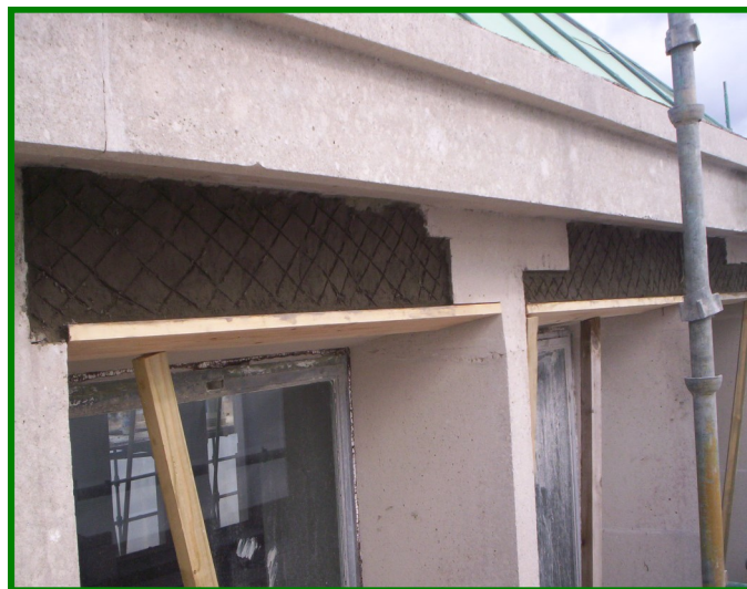
After steel treated first layers of repair mortar placed and 'scratched' ready for next layer.
