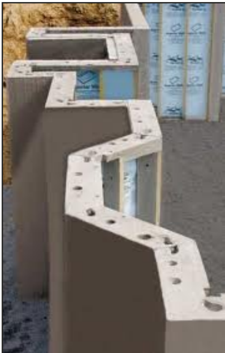
By using formwork and shuttering complicated shapes and angles be formed.
