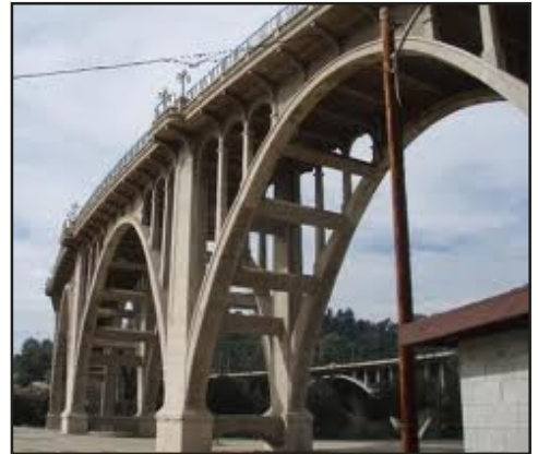
Example of Precast concrete sections used to form the deck and arches of bridges.
